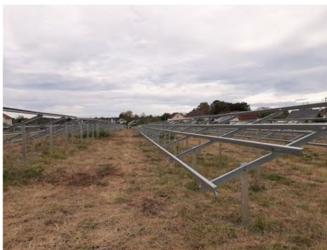
Ancrages des structures (Sources : Apex Energies)
